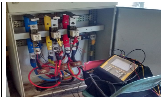
Power Measurement using Power Analyser
