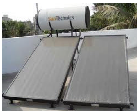
Image 9: Solar Water Heating System
